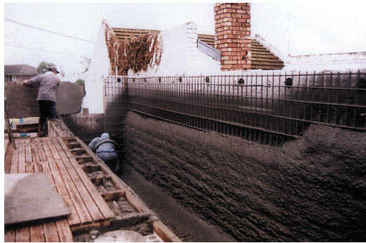
As in this second floor swimming pool, reliable waterproofing prevents leakage from tanked structures into adjacent usable space
